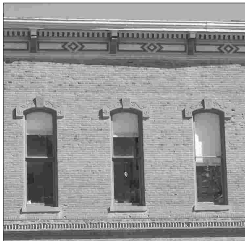
Historic window arrangements in upper stories had rhythmic patterns and typically more wall surface than windows.
