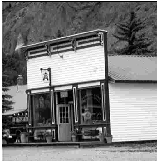
The storefront on this new building on Silver Street has the traditional arrangement of display windows and a centered entrance.
