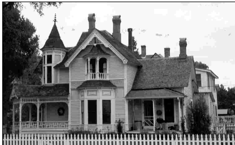
Multiple gables, bay windows, a turret, and ornate woodworking identify this residence as Queen Anne style.
