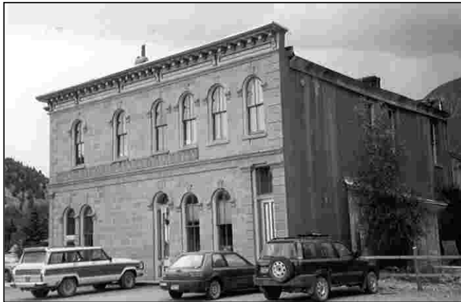
The Bank Block has a flat roof, with a parapet and roof cornice that projects above the facade roofline. Preserve historic architectural features like these.
